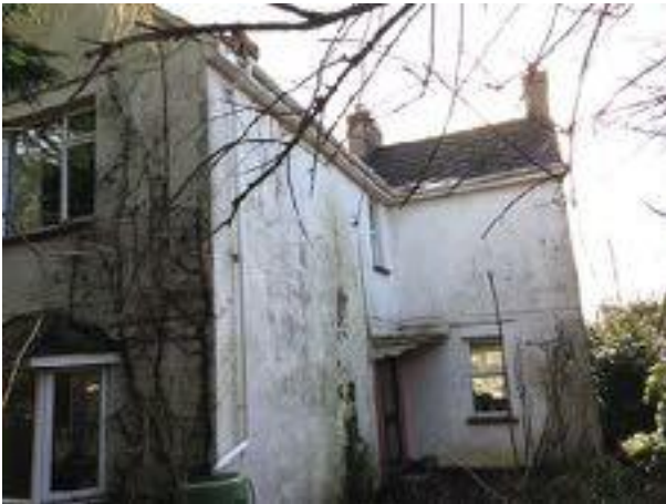
Figure 1 - Part of north and west elevations
