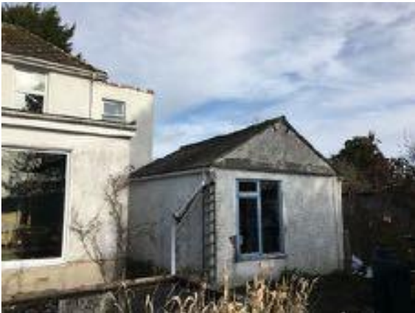
Figure 5 - Part of south and west elevations of house
