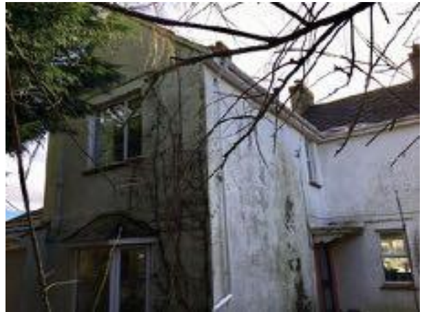
Figure 2 - Part of north and west elevations
